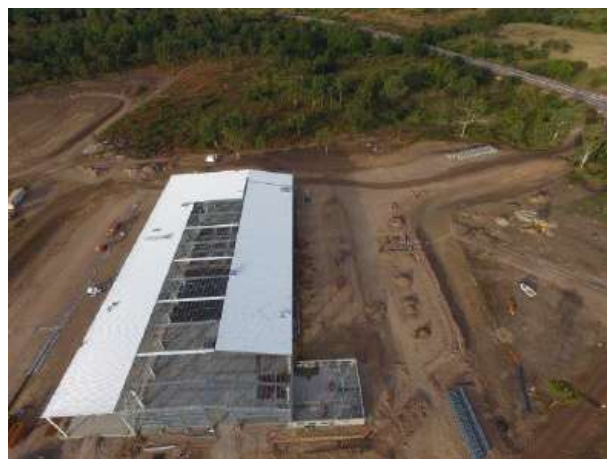
Construction stage of the Freight Distribution Centre
