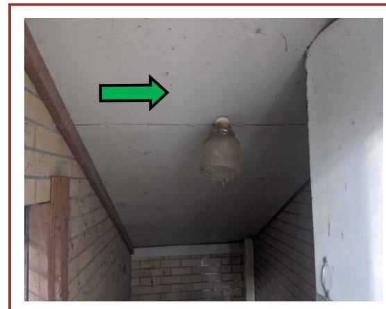
Photo #12 Internal –Ground to basement level Stairs Ceiling panels Fibre cement No asbestos detected
