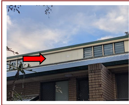
Photo #14 External –Roof level Perimeter of skylight Infill panels to windows Asbestos fibre cement
