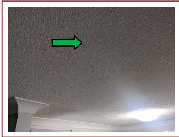
Photo #13 Internal –Level 2 Ceiling of unit 8 Textured decorative coating No asbestos detected
