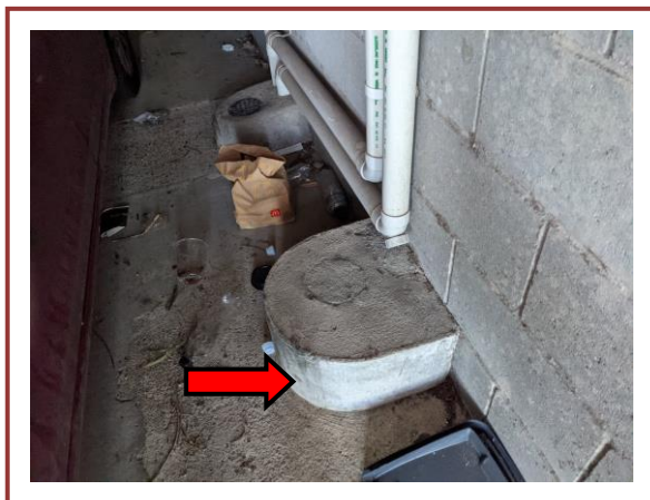
Photo #1 Internal –Ground level Garages 1,2,4 & 8 Drain trap surrounds Asbestos fibre cement
