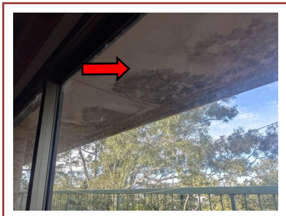
Photo #10 External –Level 3 Eat and West elevations. Soffit panels Asbestos fibre cement
