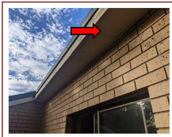
Photo #11 External –Level 3 Eat and West elevations. Soffit panels Asbestos fibre cement
