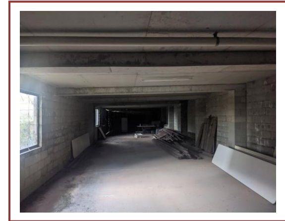
Photo #15 Internal Basement level storage No asbestos identified
