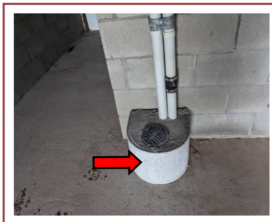
Photo #2 Internal –Ground level Garages 1,2,4 & 8 Drain trap surrounds Asbestos fibre cement
