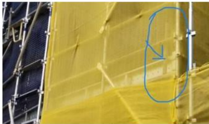
Example of short scaffold tube preventing accidental dislodgement of kickboard
