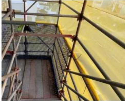
Example of Stretcher Stair with Uni-mesh on the inside landing and shade cloth to the outside
