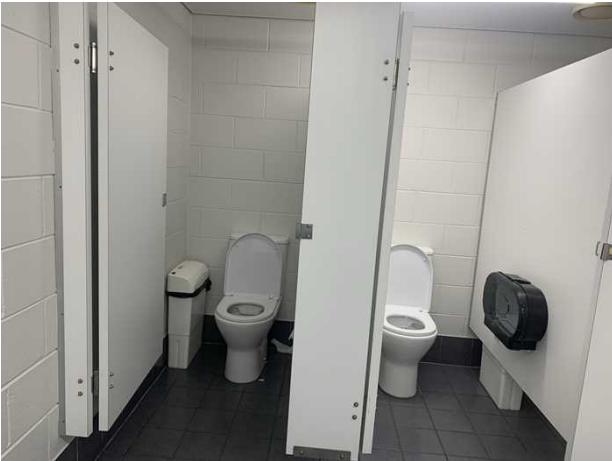
Photo 5 - Details Toilets replaced and toilet roll holders
