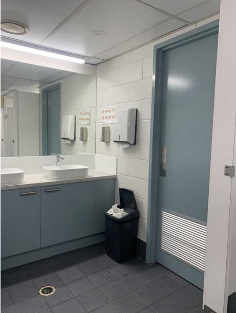
Photo 8 - Details Door vent installed
