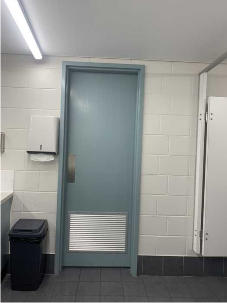
Photo 4 - Details Door vents installed
