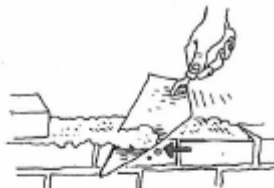
Scrape off the surplus mortar
