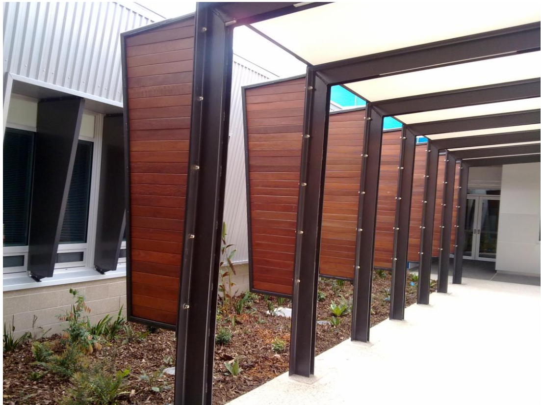
Timber 'fins' attached to the walkway columns
