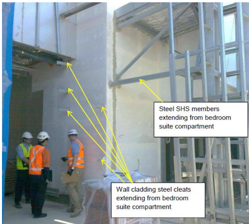
Figure 14.3 Item 1 photo steel member penetration through fire walls in IPU 3 (similar for IPU 3)
