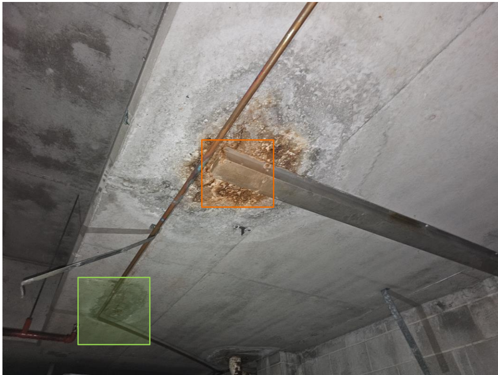
PHOTOGRAPH 9.: Defect Class B: Moderate strain to concrete, large crack at drip tray join
