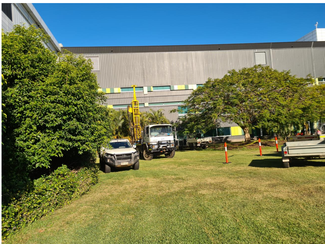
Figure 2.1 East Facing toward BH01 Location.
