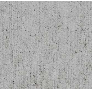
Broom finished concrete, driveway
