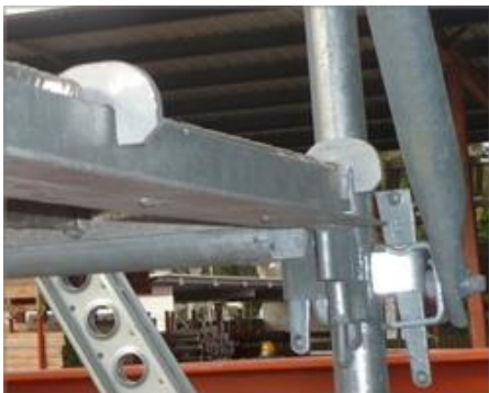
Lock hooks over the transom (Atpac Builder stairs)
