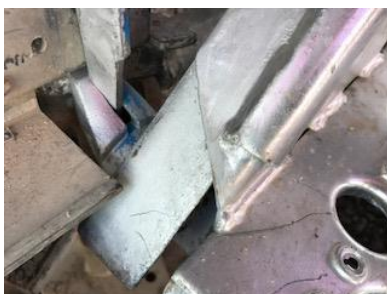
Lock hooks over the transom (Atpac Builder stairs)
