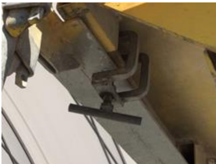
Clamp securing module to transom
