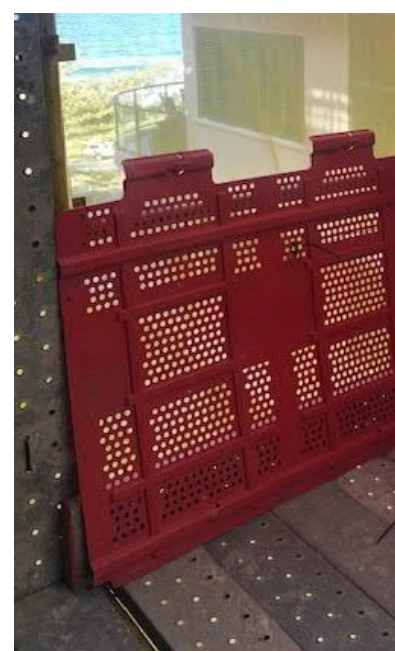
Example of ScaffoldGuard installed in front of a kickboard
