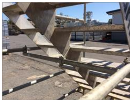
Horizontal tube and clip under stair module
