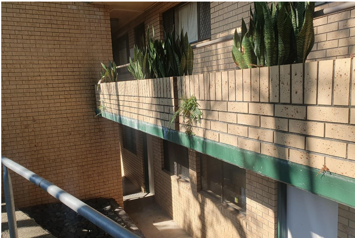
PHOTOGRAPH 2.: No evidence of concrete cancer. Efflorescence indicates on-going carbonation of concrete
