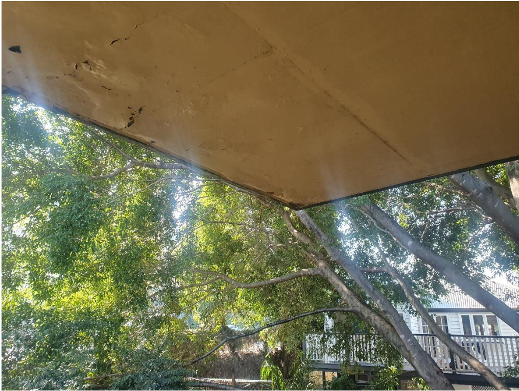
PHOTOGRAPH 19.: Corner of slab appears to be in generally good condition
