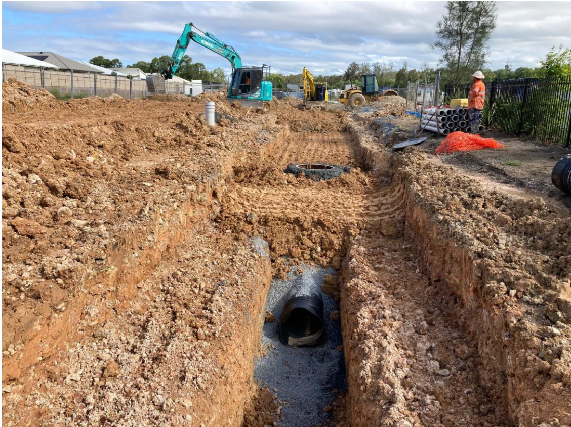
Figure 1- Stage 6 Stormwater Works
