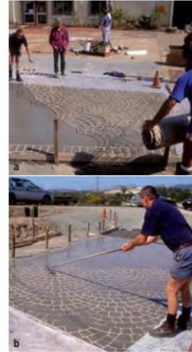
Figure 16 Placing and embedding the stencil into the 'wet' concrete [a] Border placed first [b] Stencil trowelled/rolled into surface (note plastic sheeting to protect adjoining surfaces)
