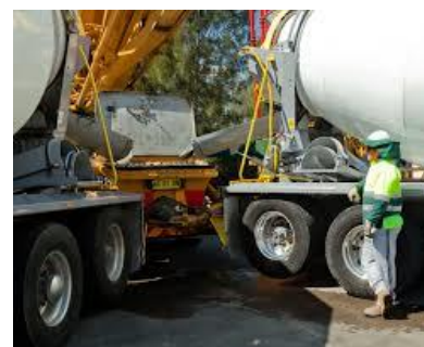
Figure 6: Concrete mixer truck filling hopper for concrete pump
