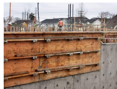
Figure 4: Concrete form work
