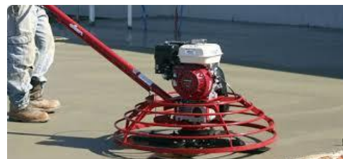
Figure 9: Concrete helicopter finisher
