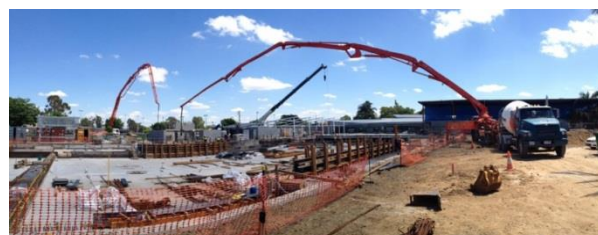
Figure 2: Concrete pumping operation
