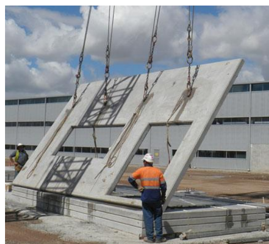
Figure 3: Tilt-up Panel being raised
