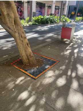
EXTENT OF TREE BASE WORK/S. 5 x 1200 x 1200MM BASES. 1 x 1500 x 2000MM BASES.
