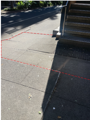
EXTENT OF CONCRETE FOOTPATH REMOVAL / REINSTATEMENT.
