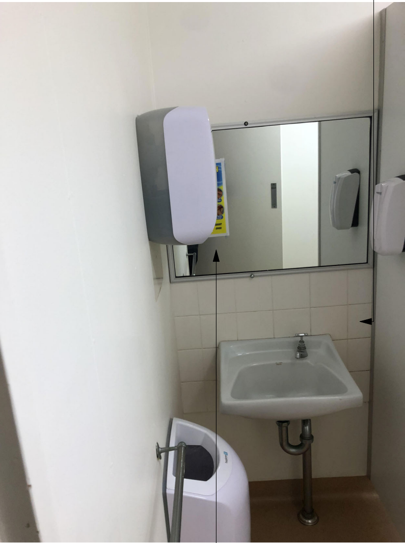
1.1 DEMOLISH EXISTING FITTINGS AND FIXTURES IN AMENITIES, CAP REDUNDANT SERVICES AND PREPARE FOR NEW.
