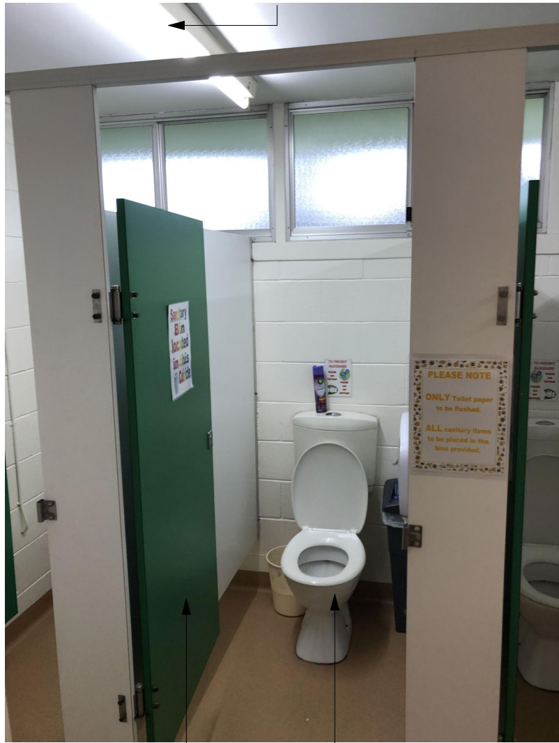
2.3 REMOVE ALL EXISTING CUBICLES REMOVE ALL FIXTURES AND FITTINGS
