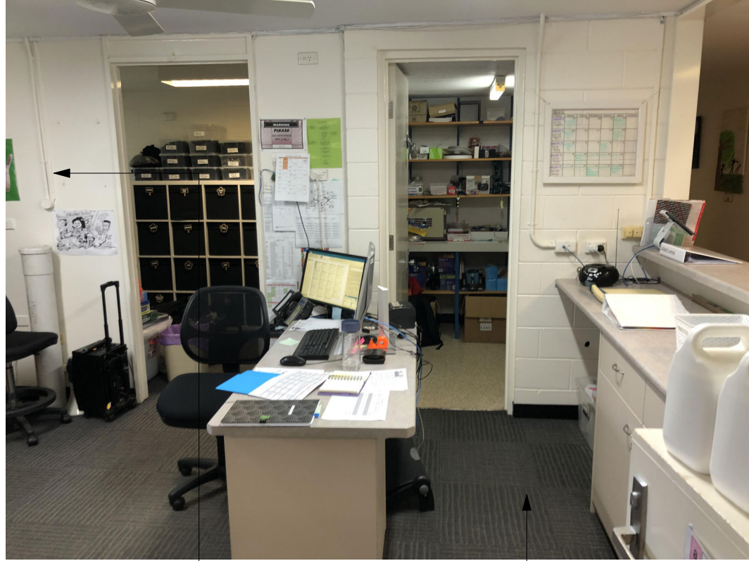
4.4 REDUNDANT CONDUITS TO BE REMOVED REMOVE EXISTING CARPET
