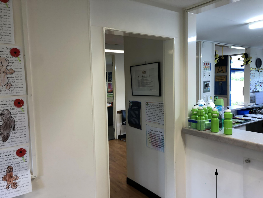
4.2 REMOVE EXISTING JOINERY
