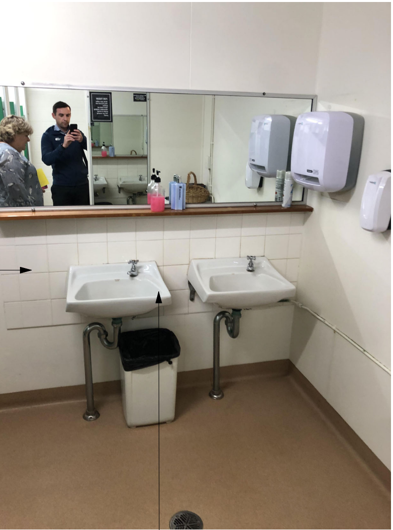
2.1 REMOVE ALL FIXTURES AND FITTINGS TO FEMALE STAFF
