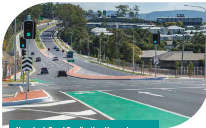
Yawalpah Road Duplication Upgrade
