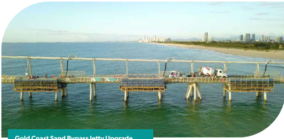
Gold Coast Sand Bypass Jetty Upgrade
