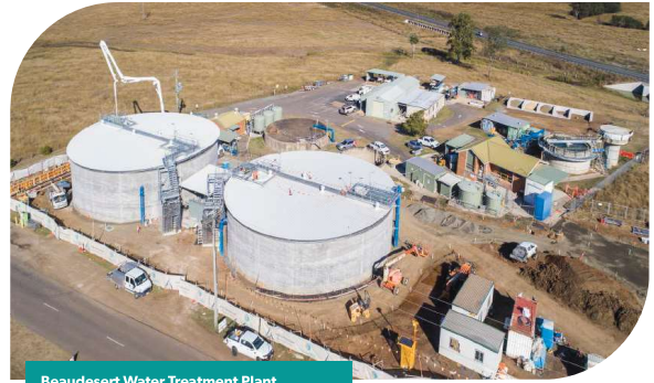
Beaudesert Water Treatment Plant
