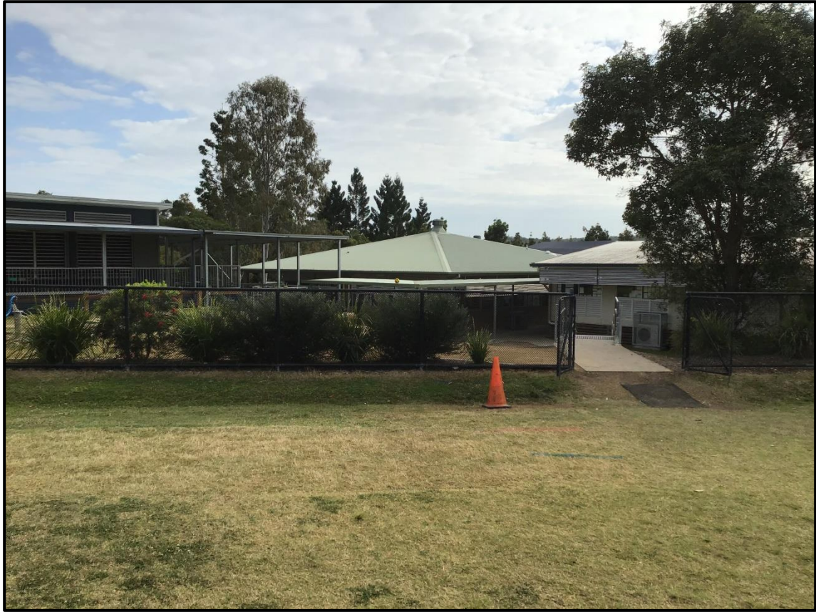
FIGURE 2 – EXISTING CLASSROOM – LOOKING NORTH
