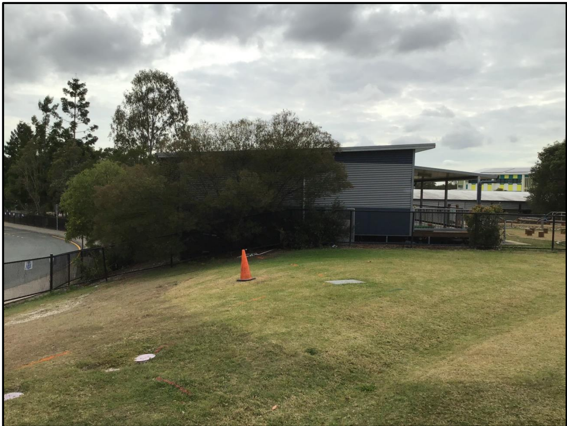
FIGURE 3 – EXISTING BATTER – LOOKING EAST
