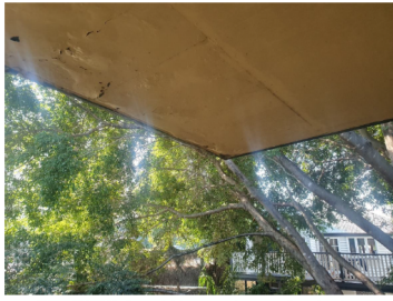
PHOTOGRAPH 19: Corner of slab appears to be in generally good condition
