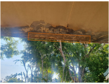
PHOTOGRAPH 12: cracking to concrete slab, spalling to some areas.
