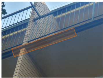
PHOTOGRAPH 41: No evidence of concrete cancer. Efflorescence indicates on-going carbonation of concrete
