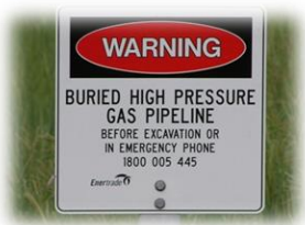
• Gas main marker
