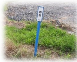
• Water main marker
