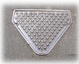
• Manhole in road
