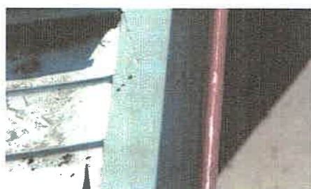
6. When the gutter has been cleaned, it should look like this.
