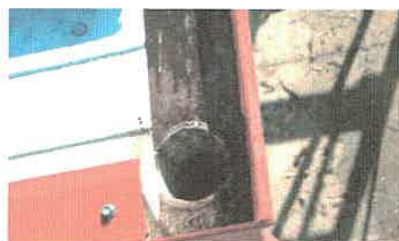
3. When litter is removed, the layer of hardened dirt is revealed below.
