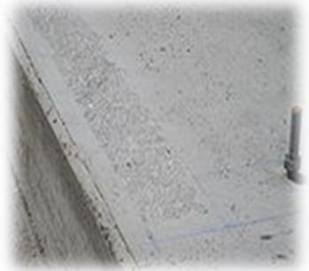
• Concrete after it has been scabbled
