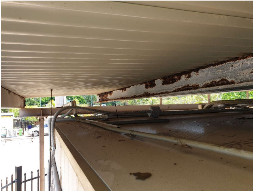
Electrical and mechanical services to existing facility
