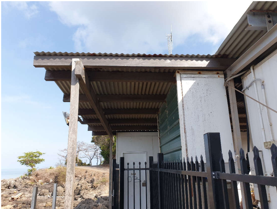
Side view of roof structure
