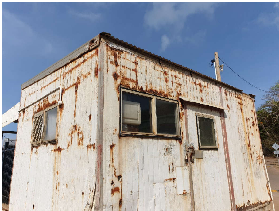
Existing Storeroom to be replaced
