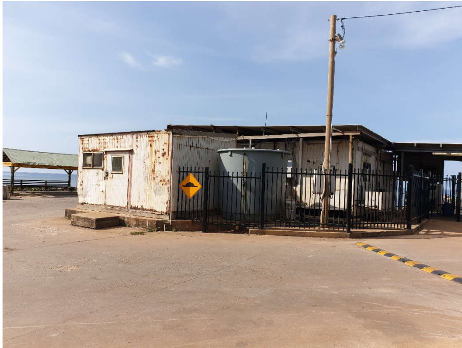
Existing Erub Community Freezer Building
