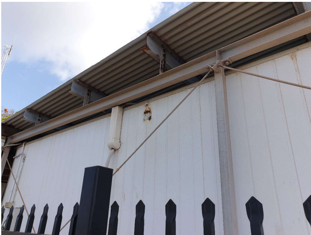
Side view of roof structure
