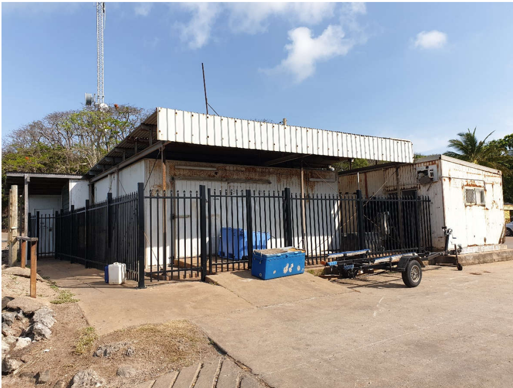
Front view of roof structure and frame to be replaced
