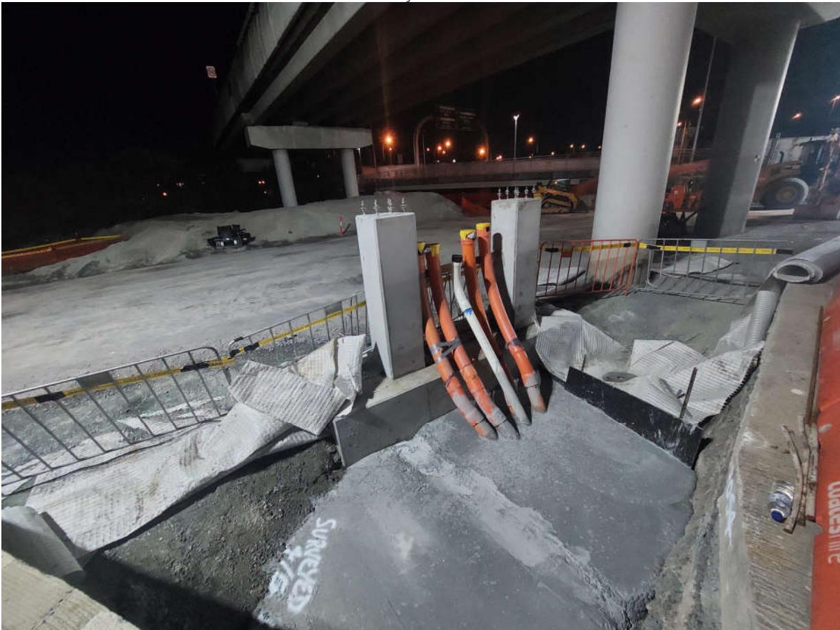
SP2 Ernie's - HDD03 Connection to Northern Gantry Columns
