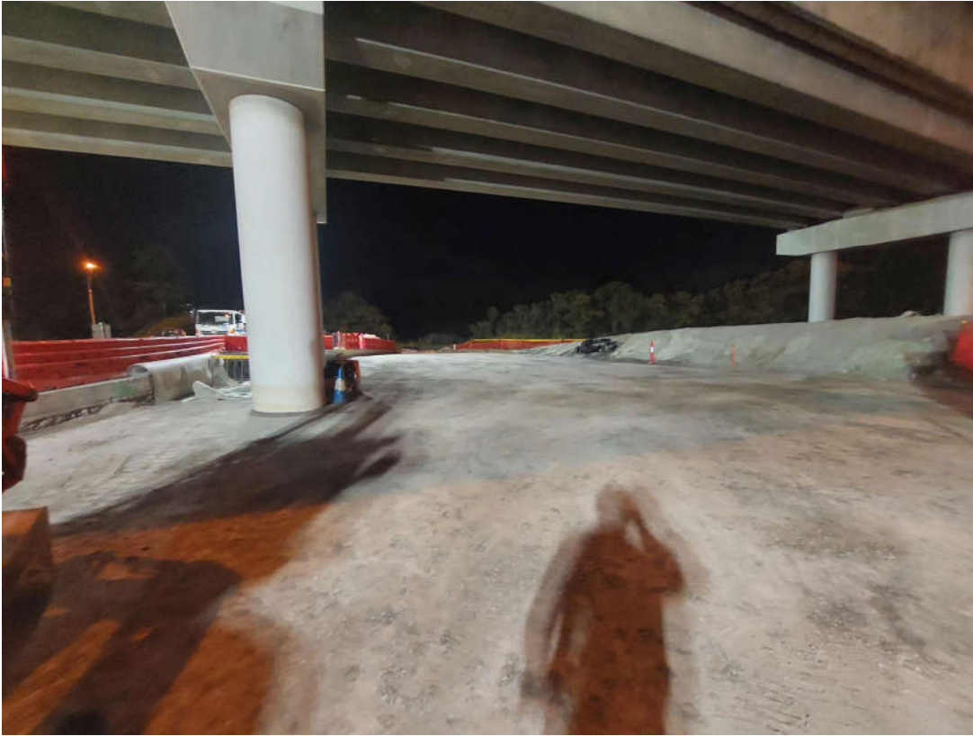
SP2 Ernie's - Northern Pavements CTB Placement
