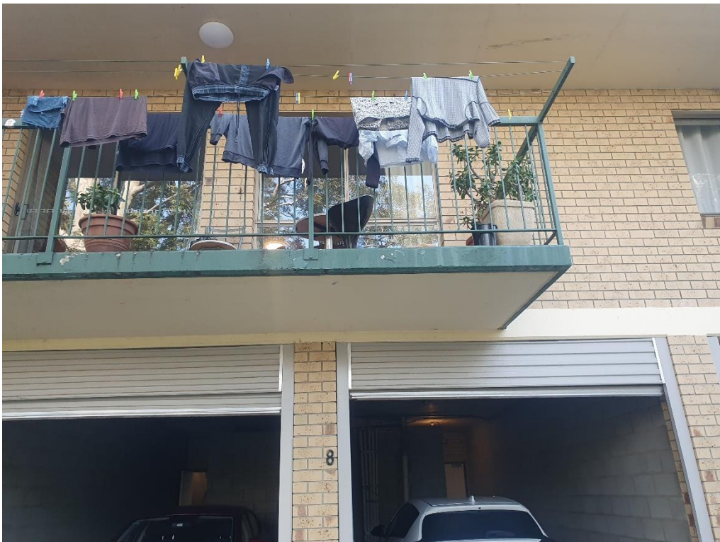
PHOTOGRAPH 28.: No evidence of concrete cancer, minor indications of deterioration. Minor defects to paint coating
