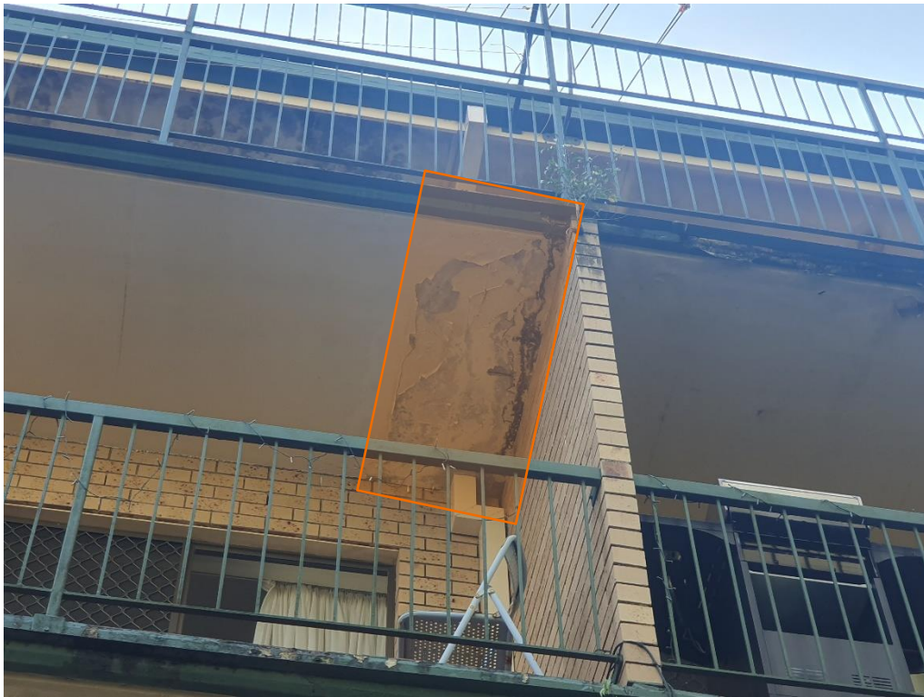
PHOTOGRAPH 43.: No evidence of concrete cancer. Efflorescence indicates on-going carbonation of concrete
