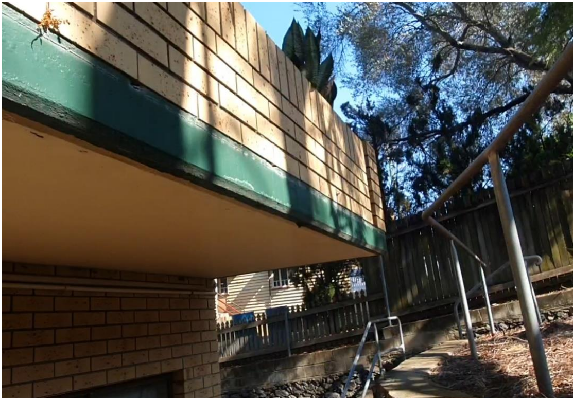
PHOTOGRAPH 1.: No evident concrete cancer, clean area of debris, clean surface & paint
