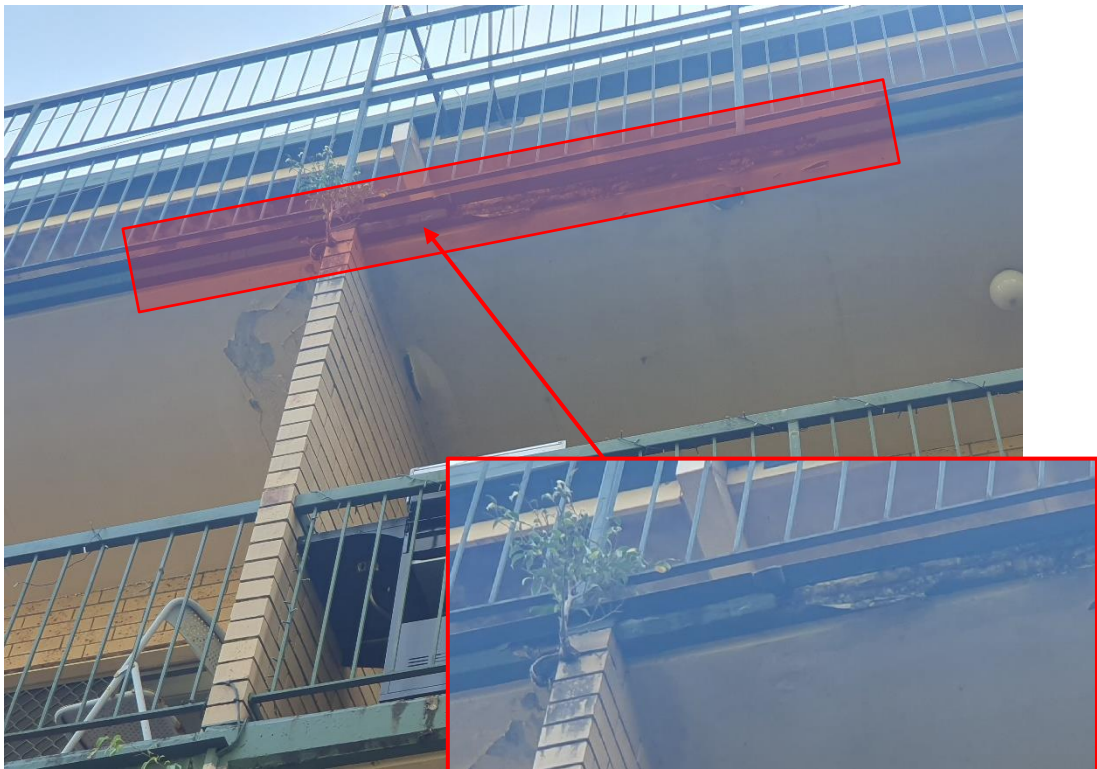
PHOTOGRAPH 42.: No evidence of concrete cancer. Efflorescence indicates on-going carbonation of concrete
