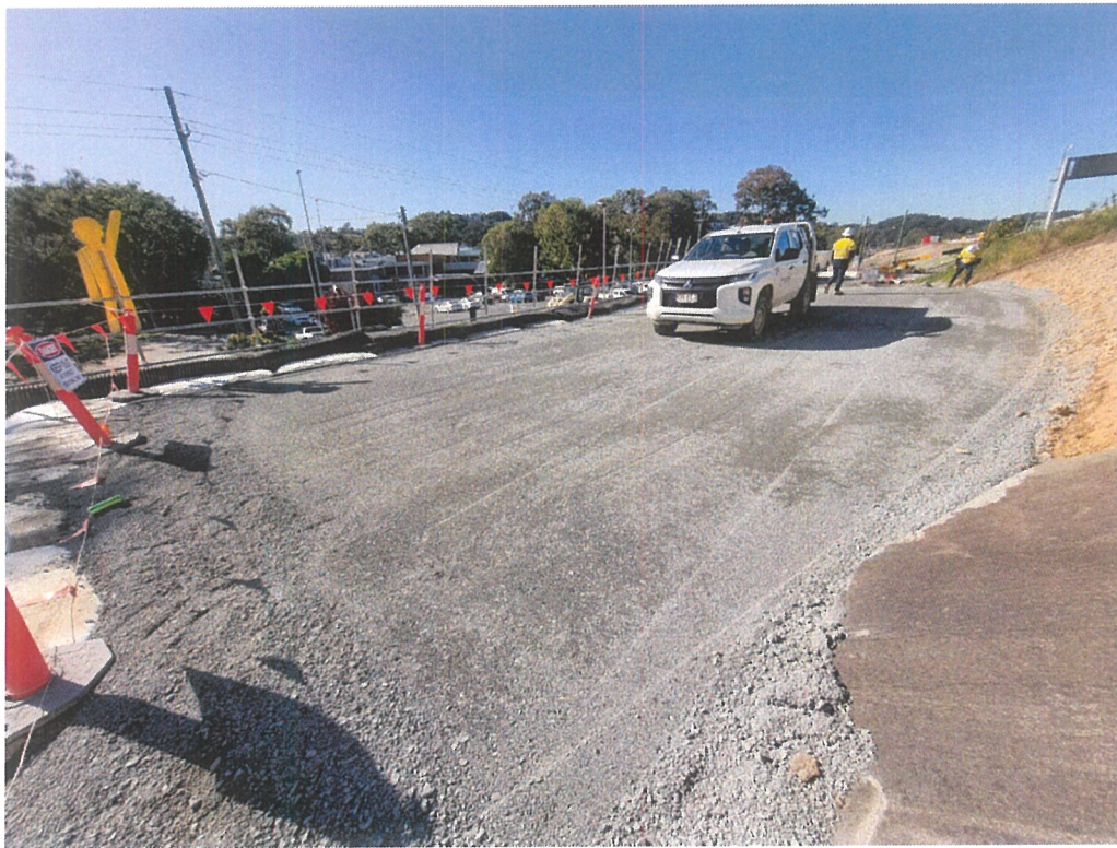
Photo 1. View of the CFA piling platform at BR07 Abut B.
